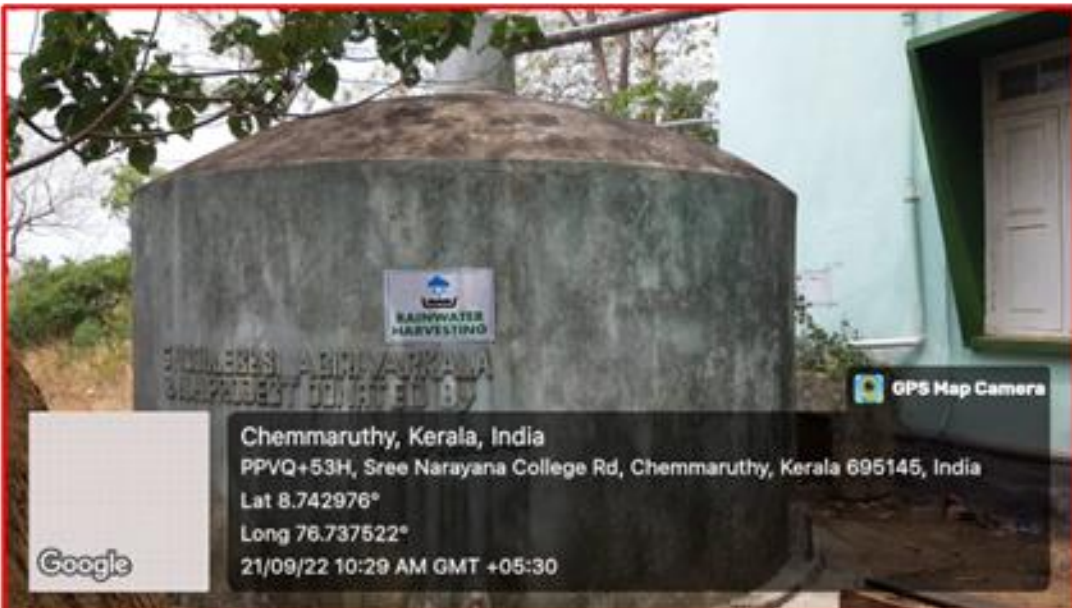
RAINWATER HARVESTING FACILITY DONATED BY PTA
